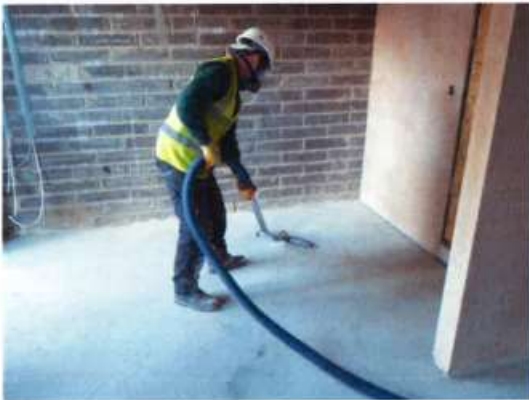
Cleaning out of plot(s)/work areas – Vacuum instead of dry sweeping wherever possible. Operative MUST also be wearing a tight-fitting face piece.
