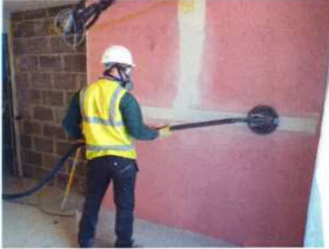
Mechanically sanding gypsum-based products – On Tool Extraction, L (Low) rated device & Operative wearing tight fitting face piece
