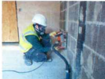
On tool extraction Wall chasing
