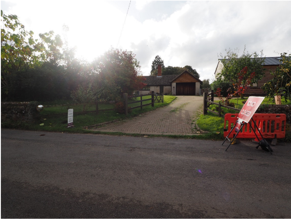
Figure 4: View of Existing Access 1 from Stone Street looking Southwest.
