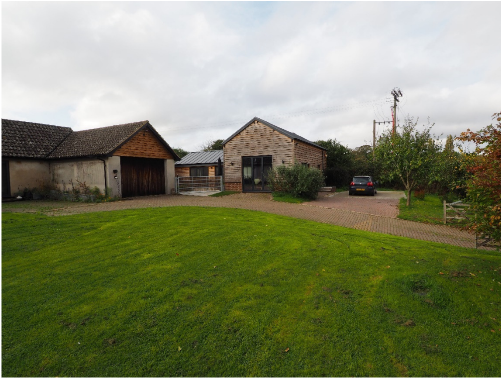
Figure 2: View of Annex from front garden looking North.
