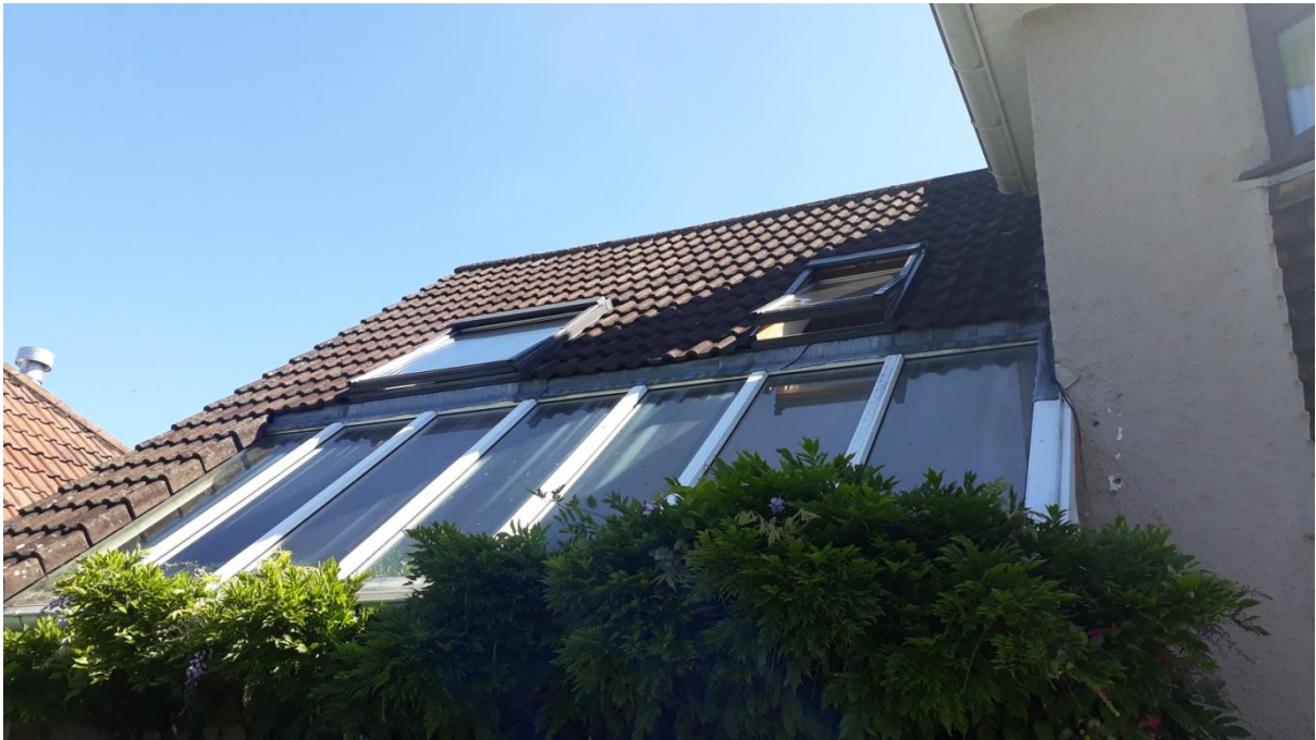
Image 2: Existing rear roof slope showing rooflights and glazing below.
