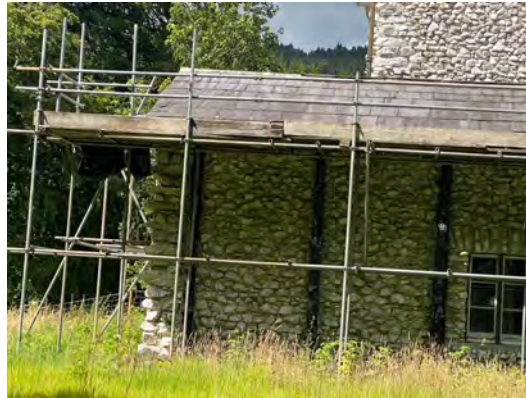
Pointed walls and slate roof.
