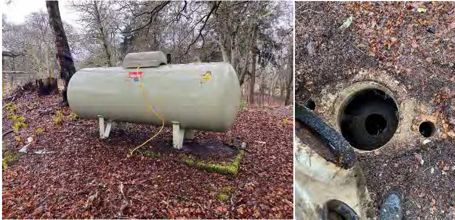
Gas and Underground Storage Tanks to rear of Dairy
