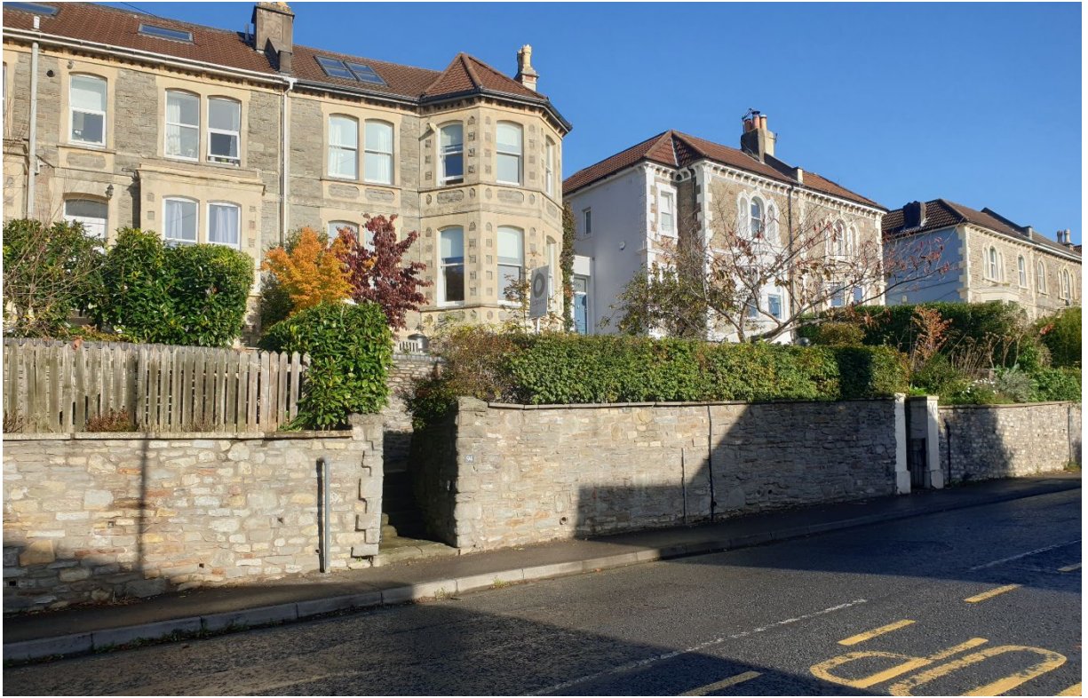
1. View from SW on Cromwell Rd.
