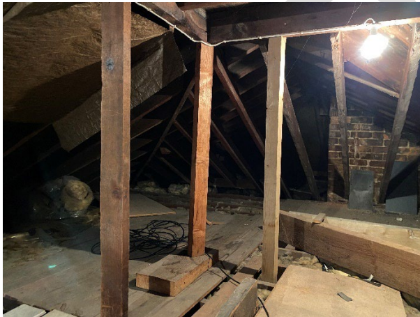
Figure 16. Internal view of the within the main dwelling.
