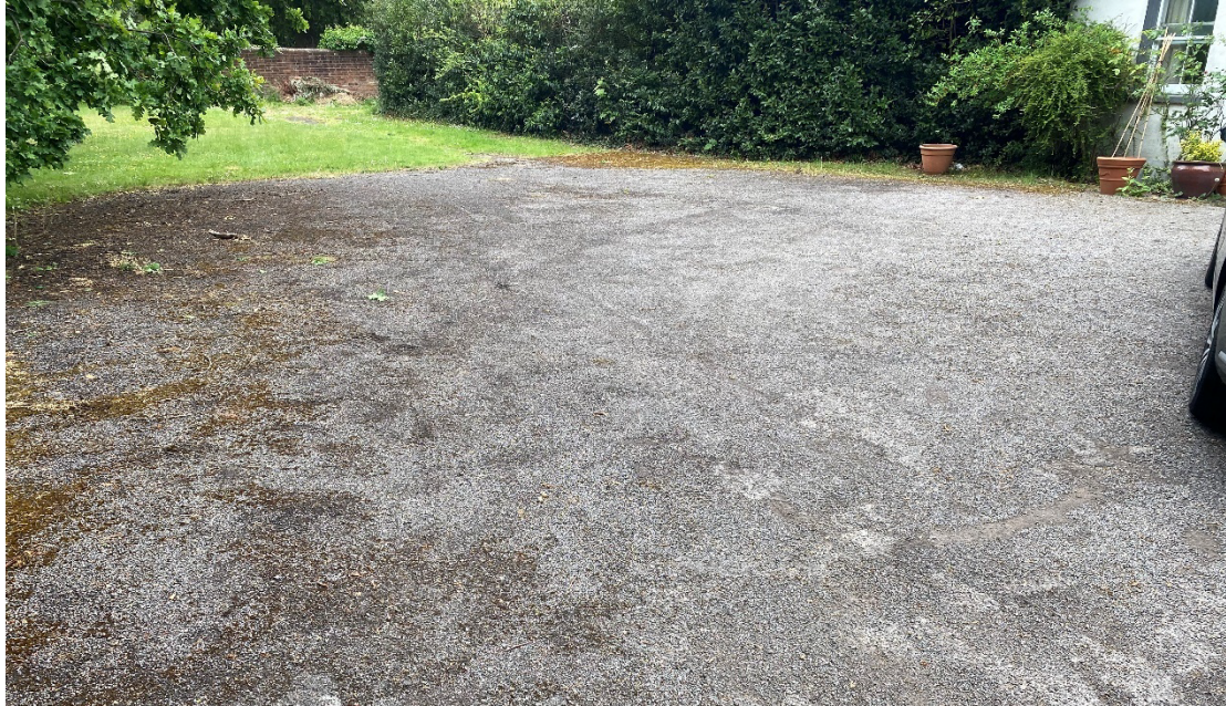
Figure 10. Hard standing driveway located to the front of the main dwelling (taken May 2022).
