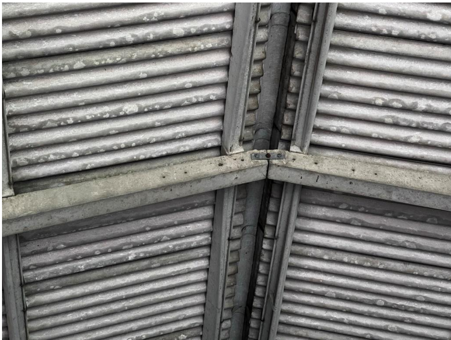
5.17 Ridge line bolted connection
