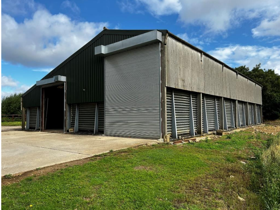
5.1 View of barn, SE corner
