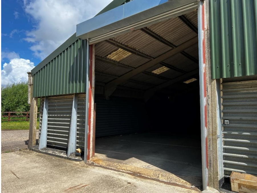
5.10 Barn internal – precast concrete portal frames spans the larger, taller area to a central column with dividing low level wall line
