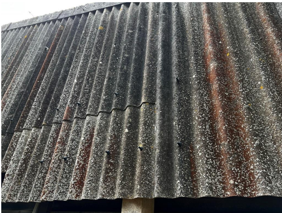
5.6 High level cladding in corrugated asbestos cement sheet
