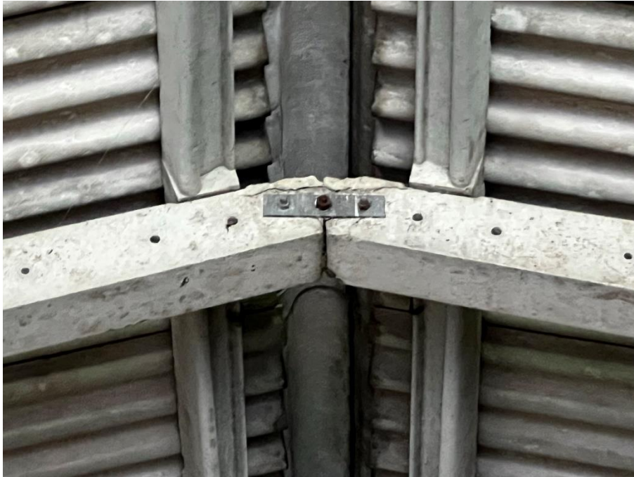
5.18 Ridge line connection – possible cracking
