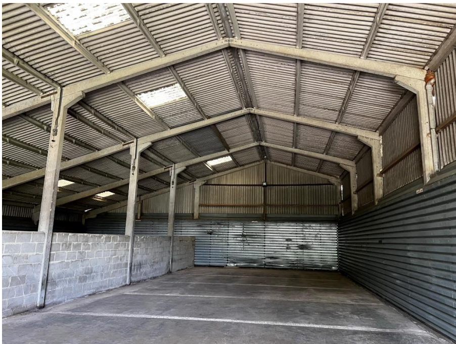
5.10 Barn internal – precast concrete portal frames spans the larger, taller area to a central column with dividing low level wall line
