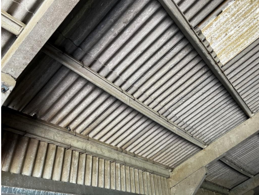
5.14 Portal bolted haunched eaves connection at west elevation
