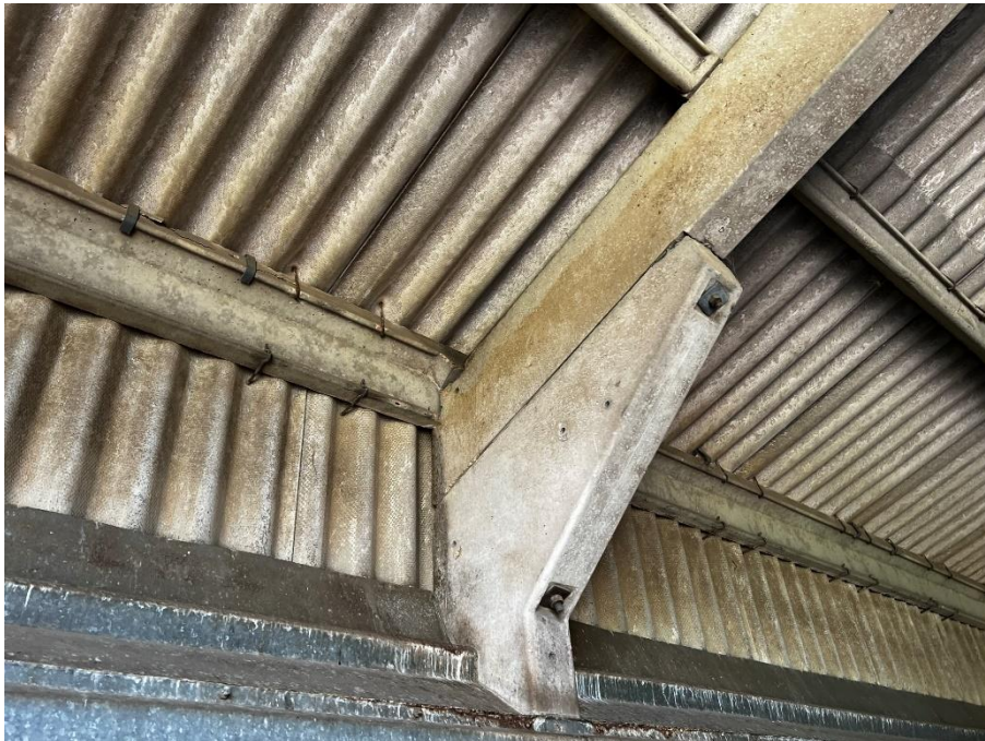
5.14 Portal bolted haunched eaves connection at west elevation
