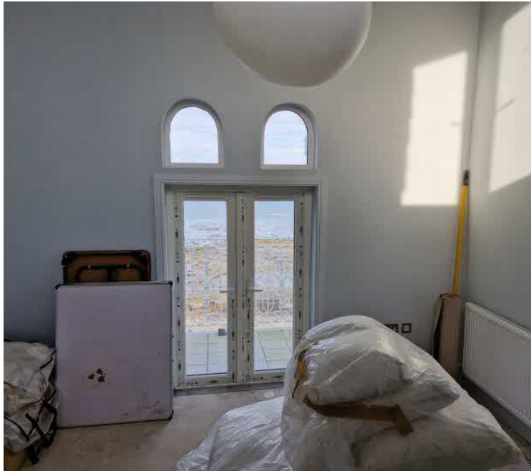
Figure 2: Internal view of front elevation existing windows/doors looking seawards
