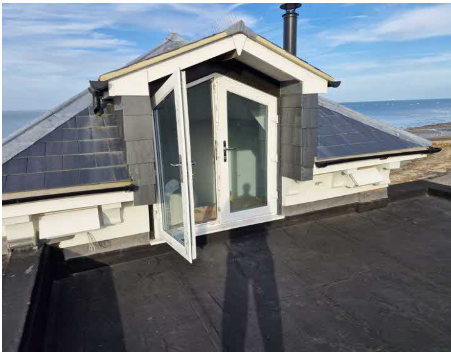
Figure 3: Existing rear roof level with existing access doors
