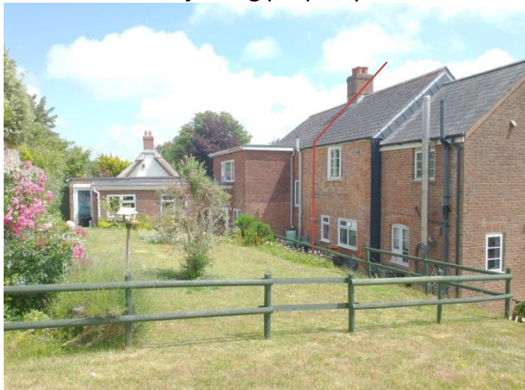
Rear elevation showing the extended adjoining property (No.20) beyond.
