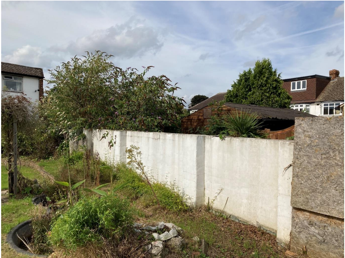
Rear looking right towards No.121
