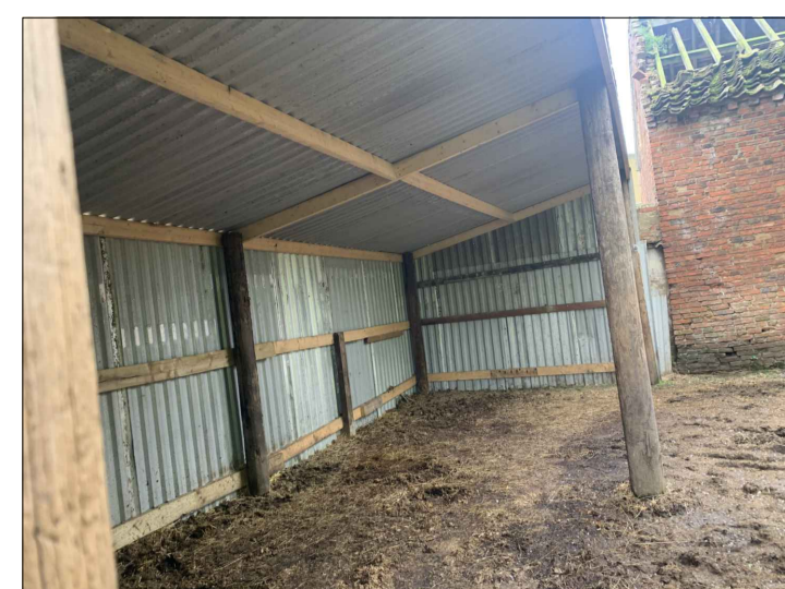
Photo 2 Existing Field Shelter 01
