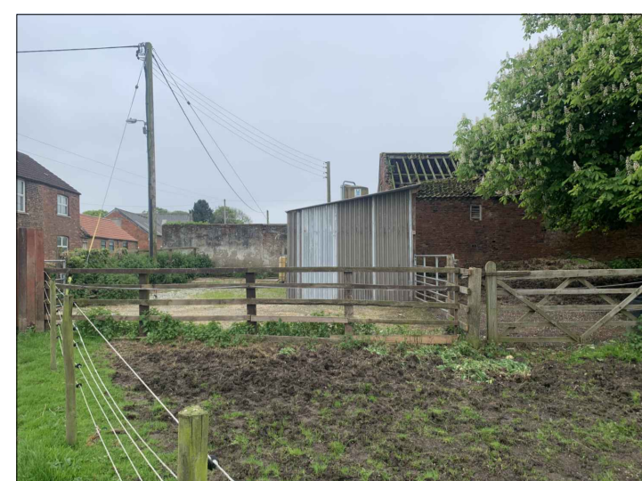
Photo 1 Existing Field Shelter 01
