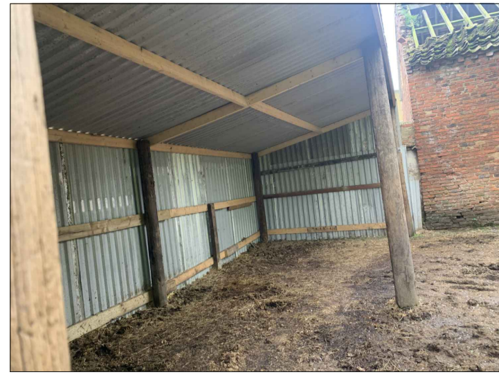
Photo 2 Existing Field Shelter 01
