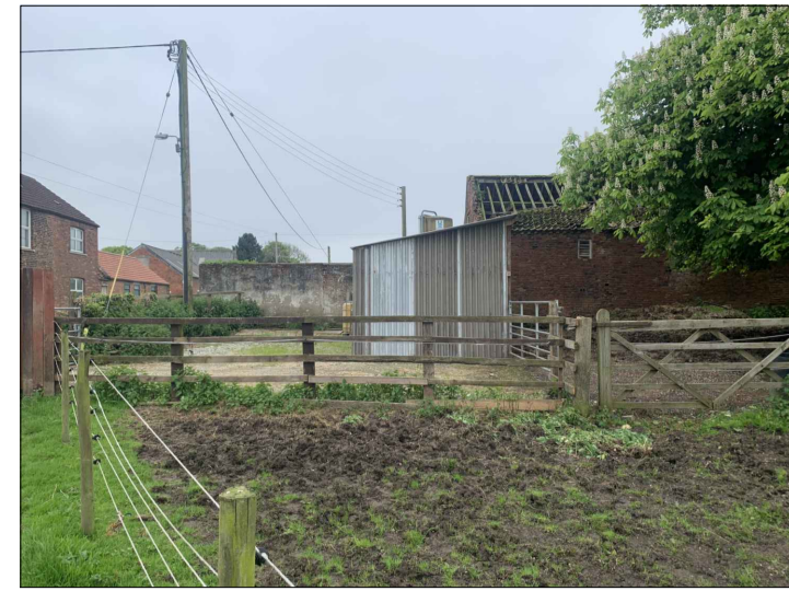
Photo 1 Existing Field Shelter 01
