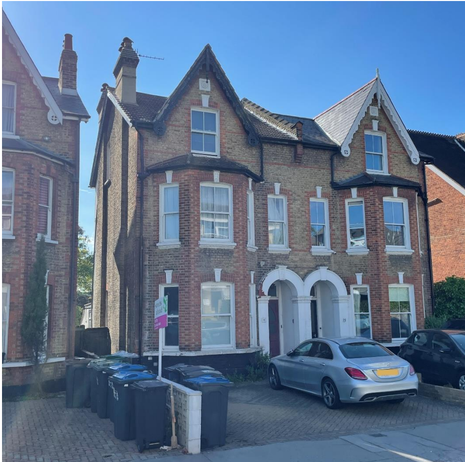
Figure 1 View of the front elevation 11 Chatsworth Road
