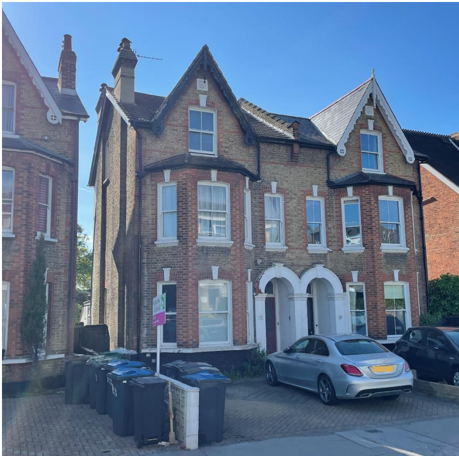
Figure 2 View of the front elevation 11 Chatsworth Road.
