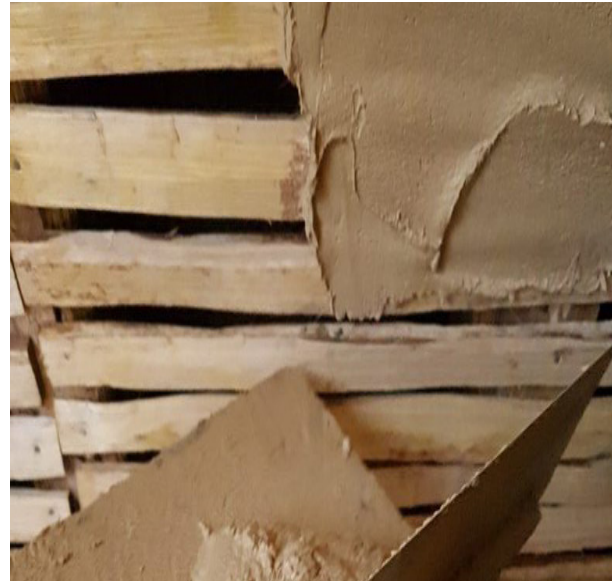
Lime plaster scratch coat
