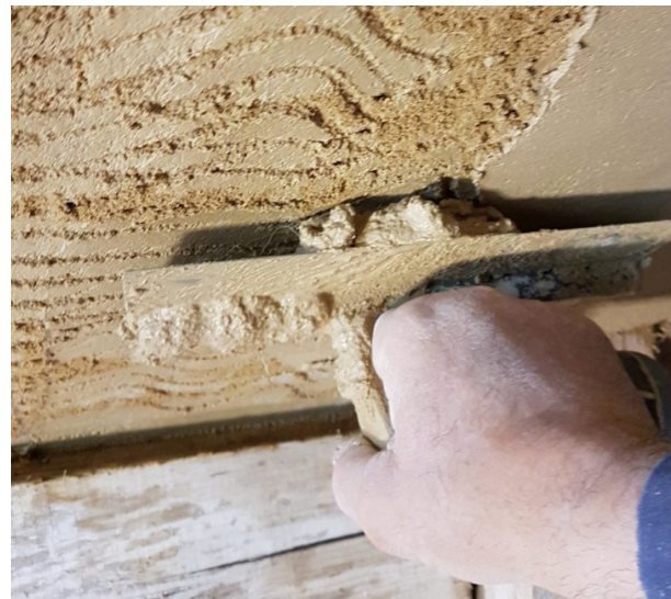
Lime plaster top coat
