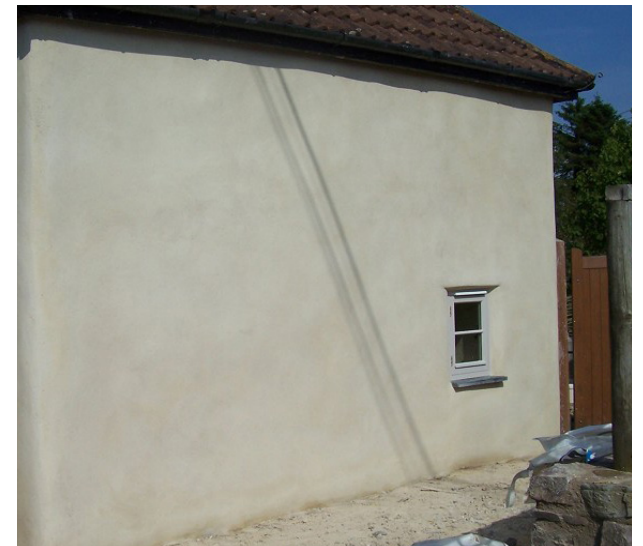
Finish coat of lime render
