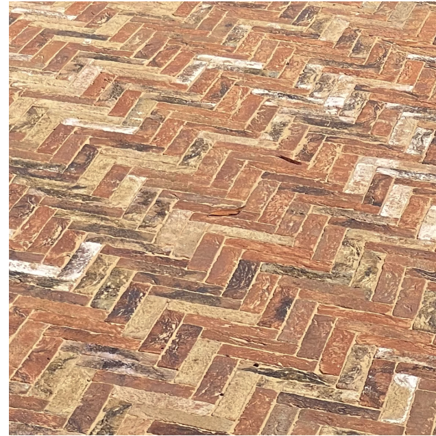
2. Paving and terracing to main garden
