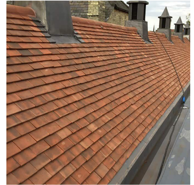
4 Annex roof tile
