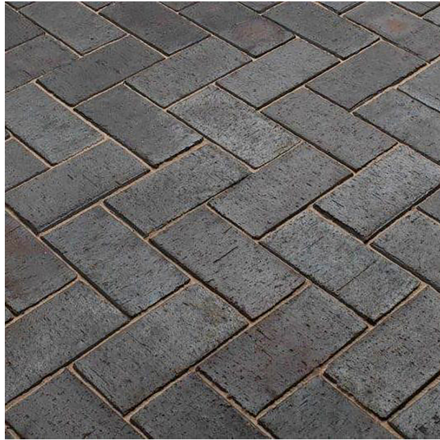
1. Paving to front of main house
