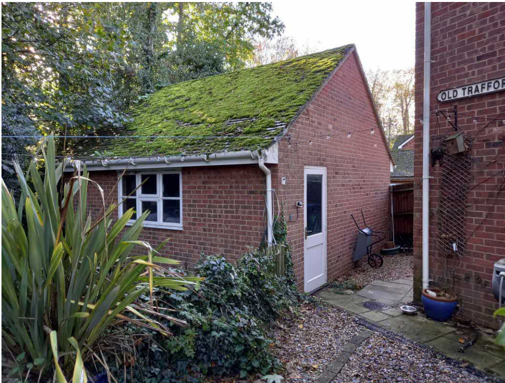
Rear elevation of existing garage
