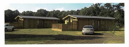
Panel cabins have the added benefit of insulation within the timber frame panel. Depending on client insulation requirements, external wall panels can be 100mm or 150mm thick with fulfill standard insulation or higher grade stecio wood fibre insulation.
