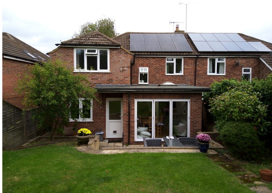
Existing rear view
