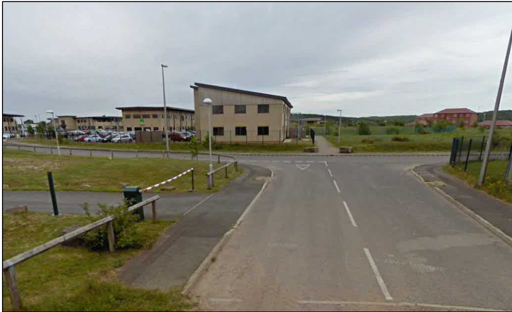
Figure 5: Existing service road at Burbank Avenue (looking east to Darwin Drive)
