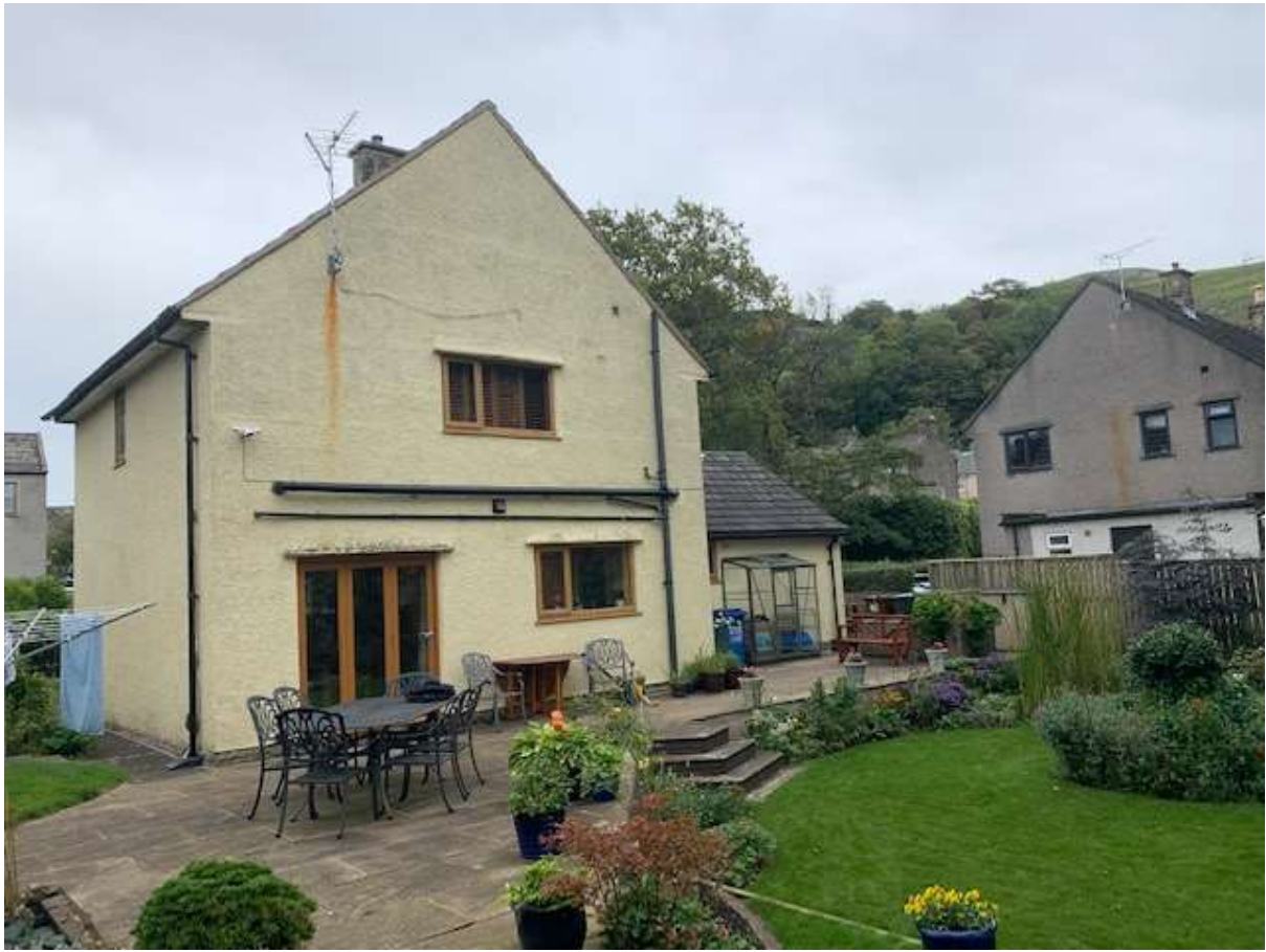
South Elevation – extension to project off the single storey extension to the east using matching materials to the host building
