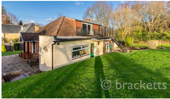
Existing bungalow - South east elevation
