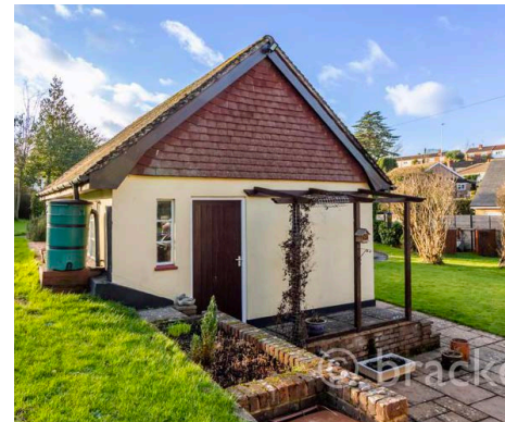
Existing garage to be removed
