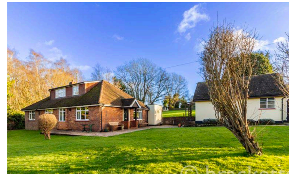
Existing Bungalow and garage, North west elevation
