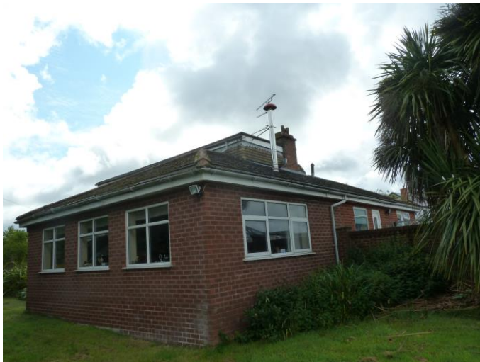
Photograph 6: B1 – typical view of the north and east (side) elevations.
