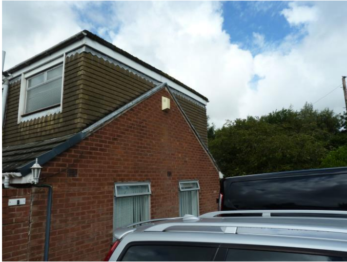
Photograph 5: B1 – typical view of the east (side) elevation.
