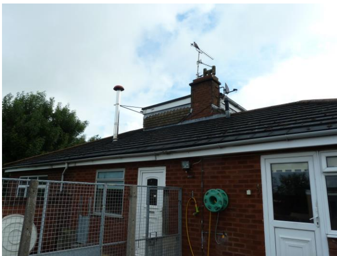
Photograph 7: B1 – typical view of the east (side) elevation.
