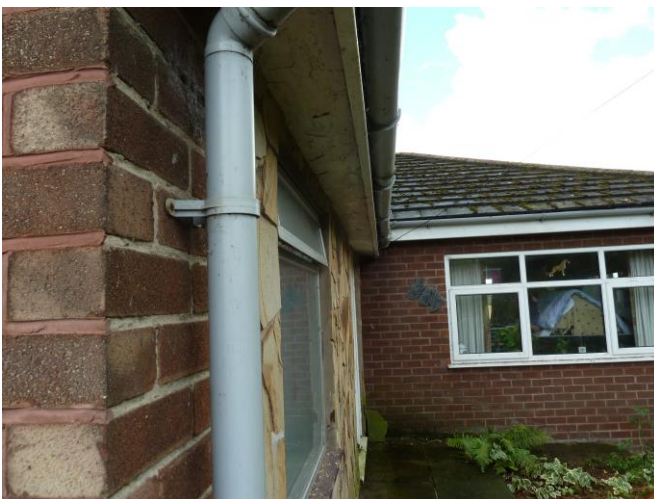
Photograph 10: B1 – front elevation looking west. Note tight fitting soffits.
