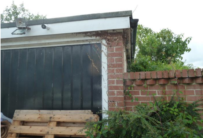
Photograph 14: B2 – typical view – flat roofed and tight-fitting door and soffits and no PRFs.
