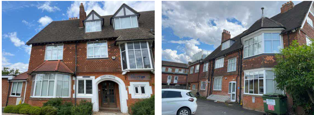
Figures 21 and 22: Front elevation existing dormers and location of new proposed dormer (left) and rear elevation flat roofed dormers proposed for replacement
