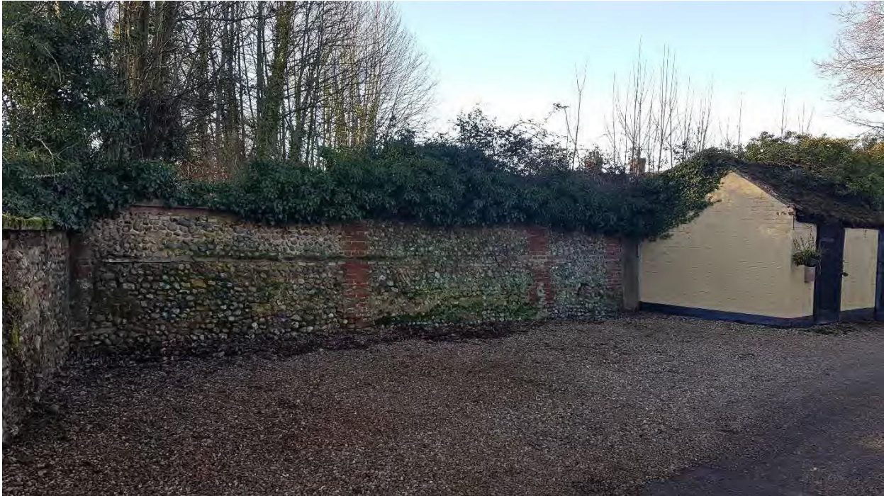
Plate 2: Boundary wall and side elevation of outbuilding.
