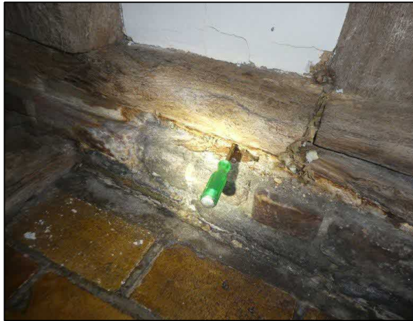
Rot to plate internally
