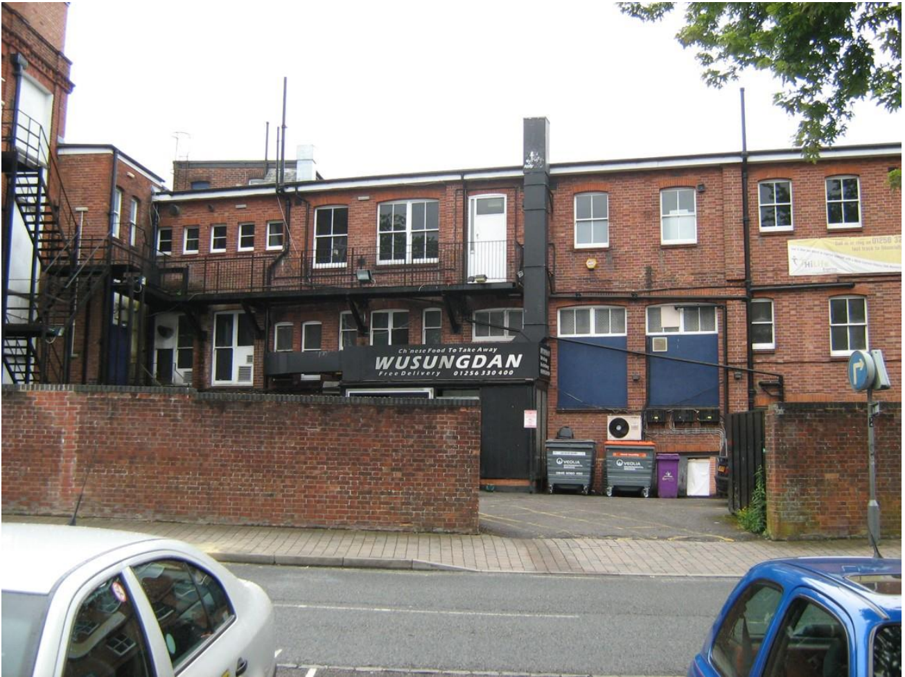
View of the north façade (Rear) of the property from Joices Yard
