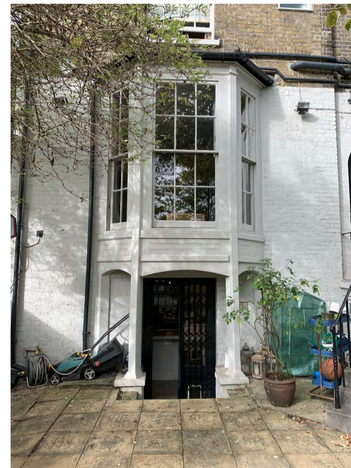
Existing rear bay window
