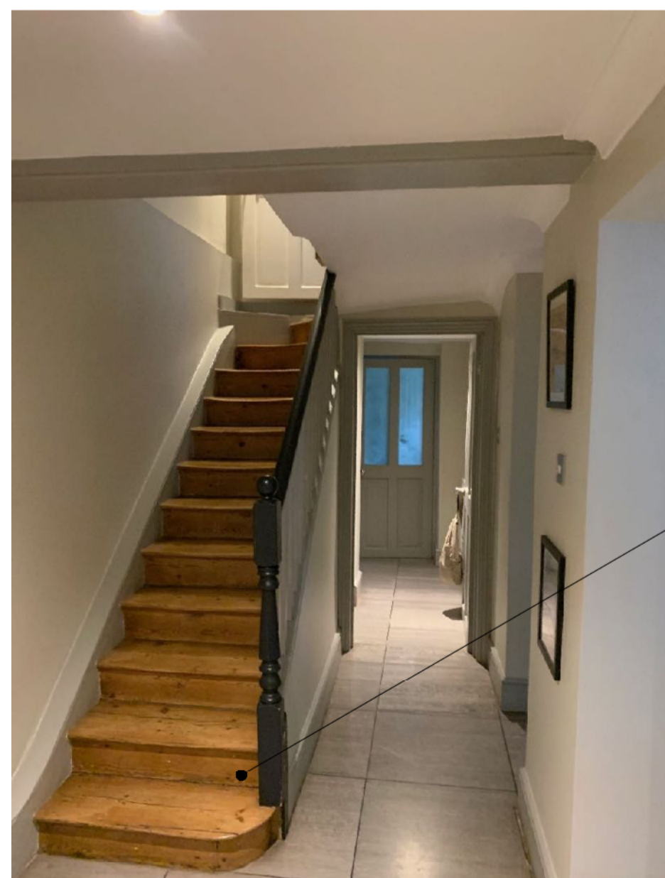
EXISTING LGF STAIRCASE
