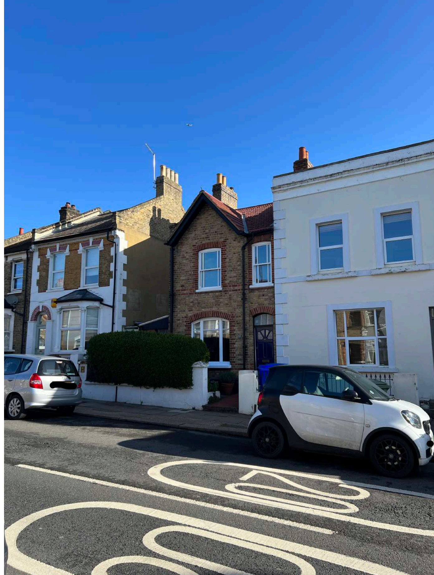
Existing front facade_35 & 41 in context
