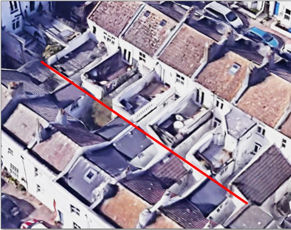
Above: Aerial view of full-length roof terraces to the rear of College Gardens with the rear boundary line indicated (© Google).
