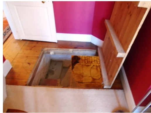
Figure 6 Existing trap door in the library, which leads down to the cellar
