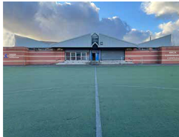
OUTSIDE Image 8 Brick Walls at pitch RCF ICC - cut out raised letters glued to wall
