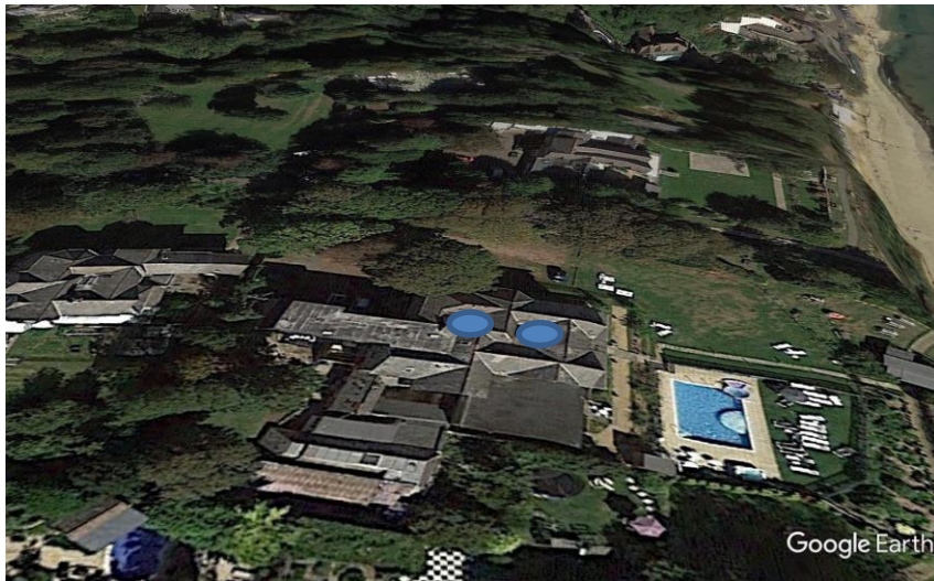
Position of bat droppings in roof space
