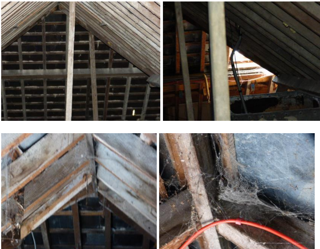
General views of the roof space
