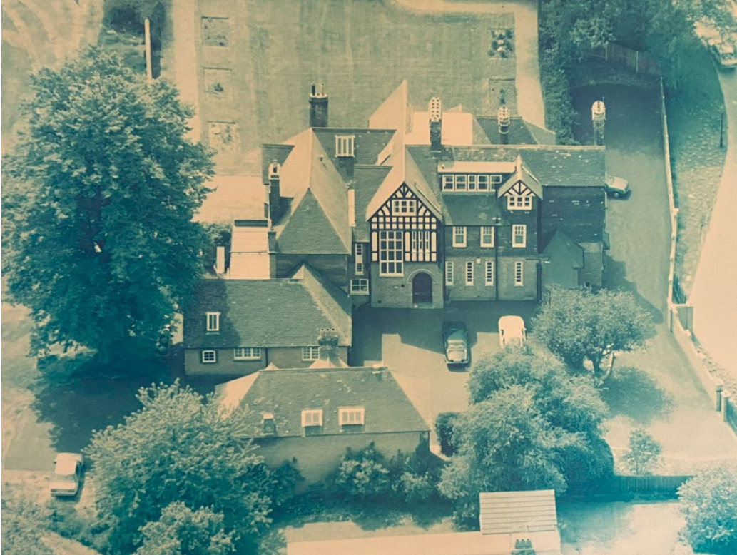
Fig. 4: Aerial Photograph c.1980s
