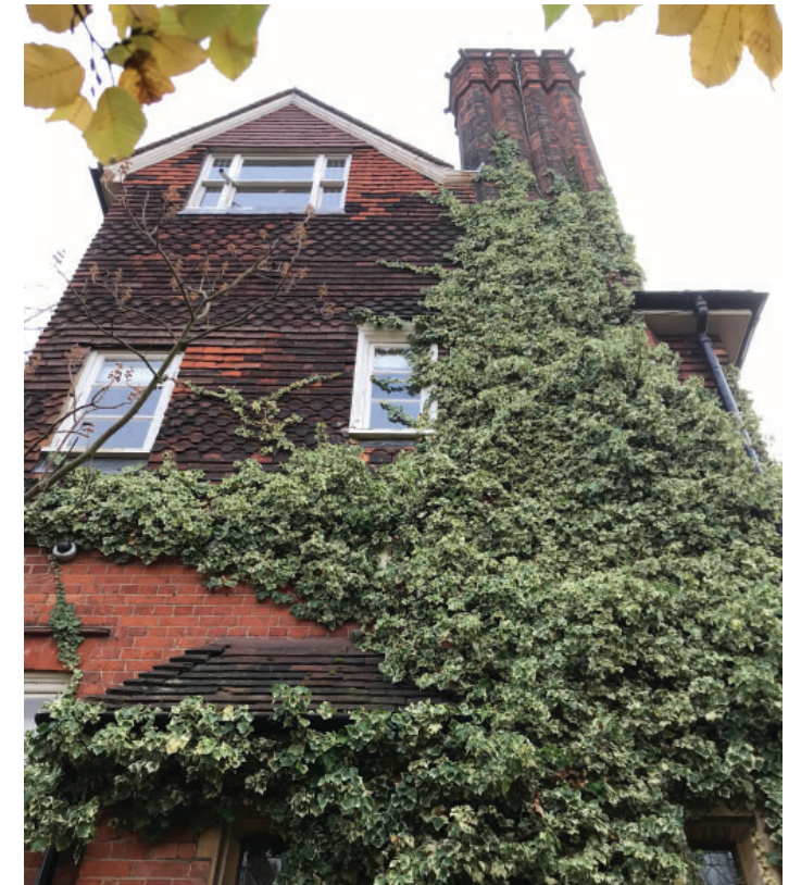
5. View of west elevation of the main house
