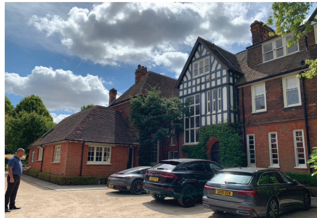
1. View of the main house from driveway
