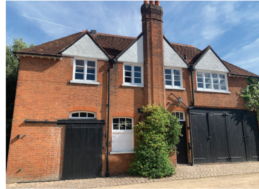
4. View of coach house from driveway
