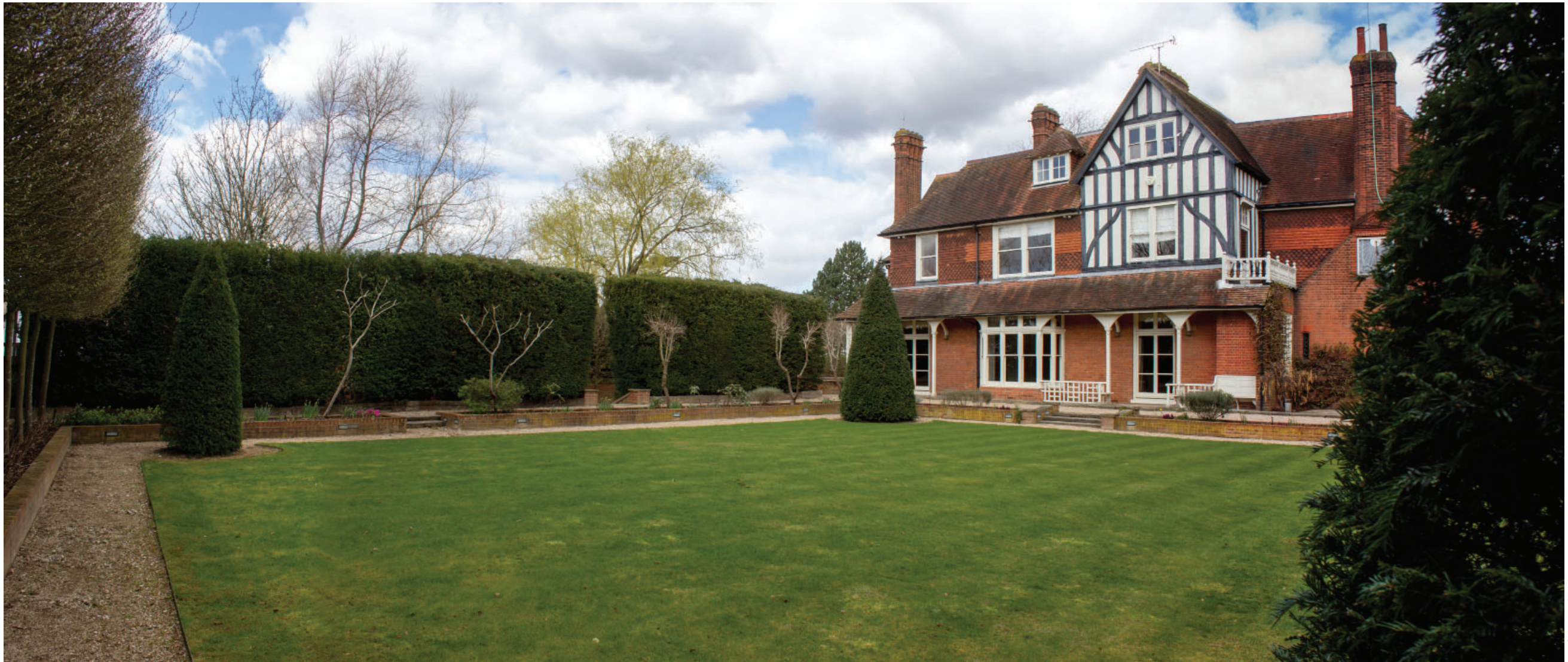
Image of south elevation showing repositioned double doors from snug.
