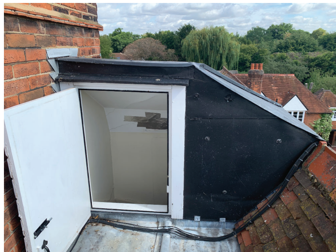
Existing access to the roof to be removed
