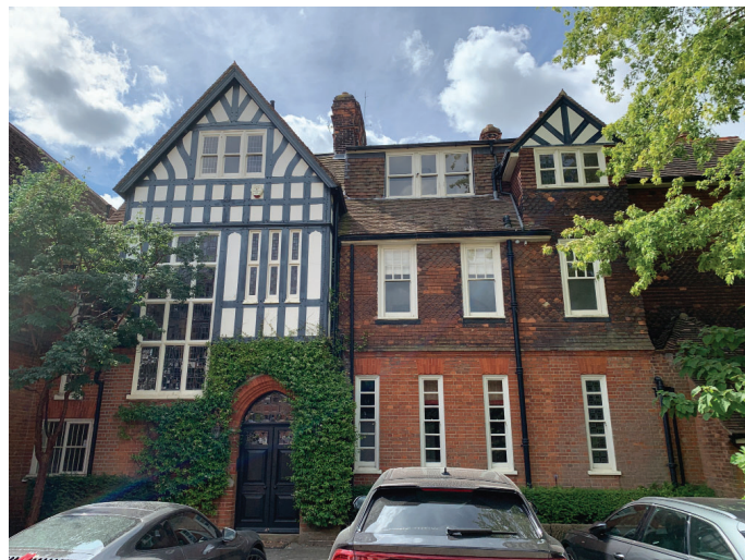
Existing North elevation showing non original dormer window
