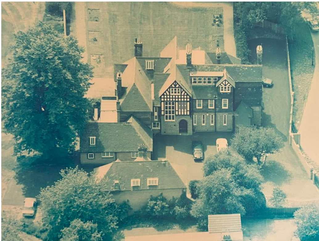
Fig. 4: Aerial Photograph c.1980s
