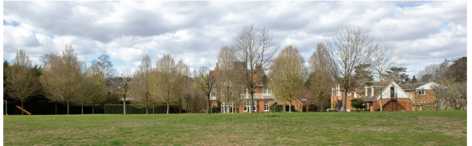
1. View of main house and ancillary buildings (including Garage) from across the green belt land.
