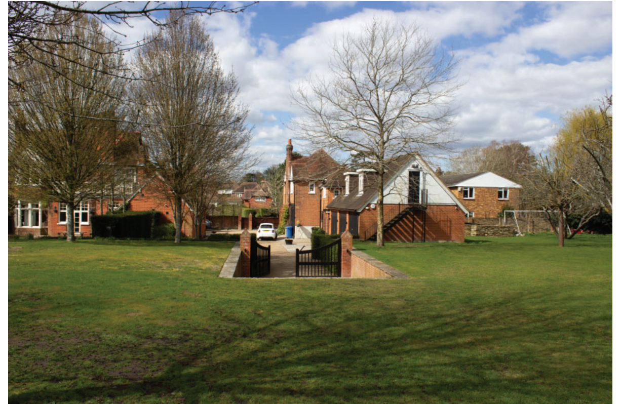
4. View of existing garage building
