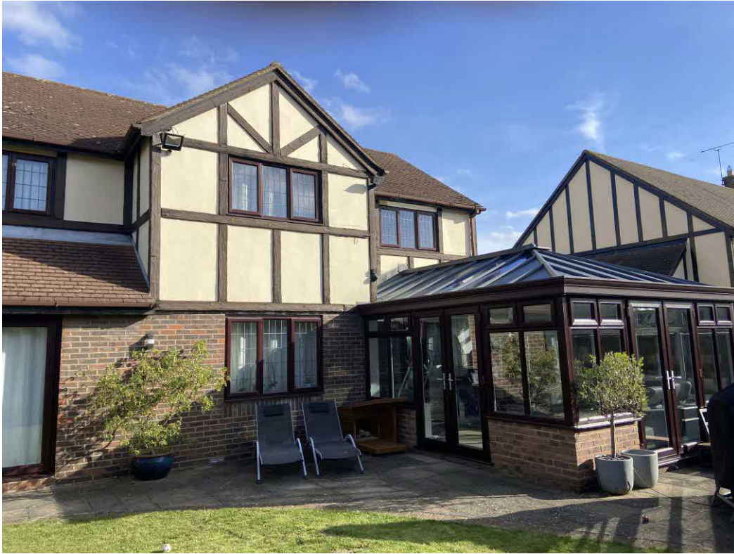
Rear elevation photo
