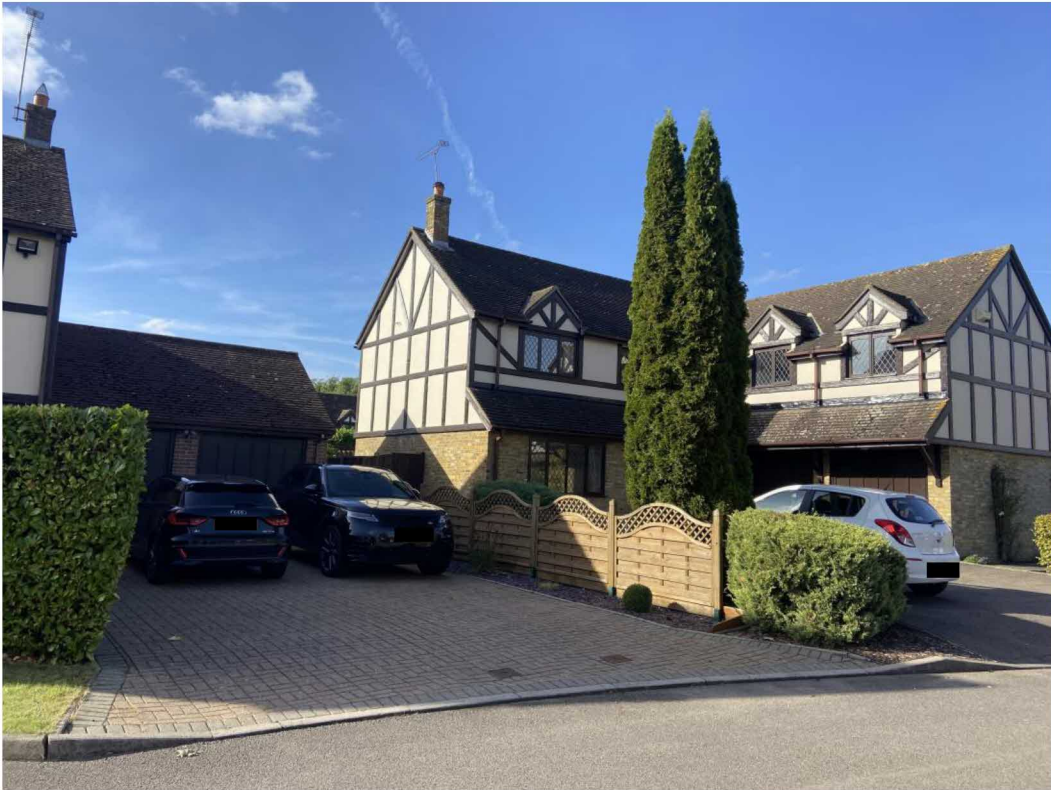
Neighbour at number 4 is displaying gable end dormers above the garage and a tiled roof overhang over the garage door. This detail has been replicated in the proposed drawings.
