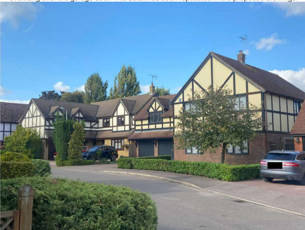
Other neighbouring properties displaying the same architectural details.
