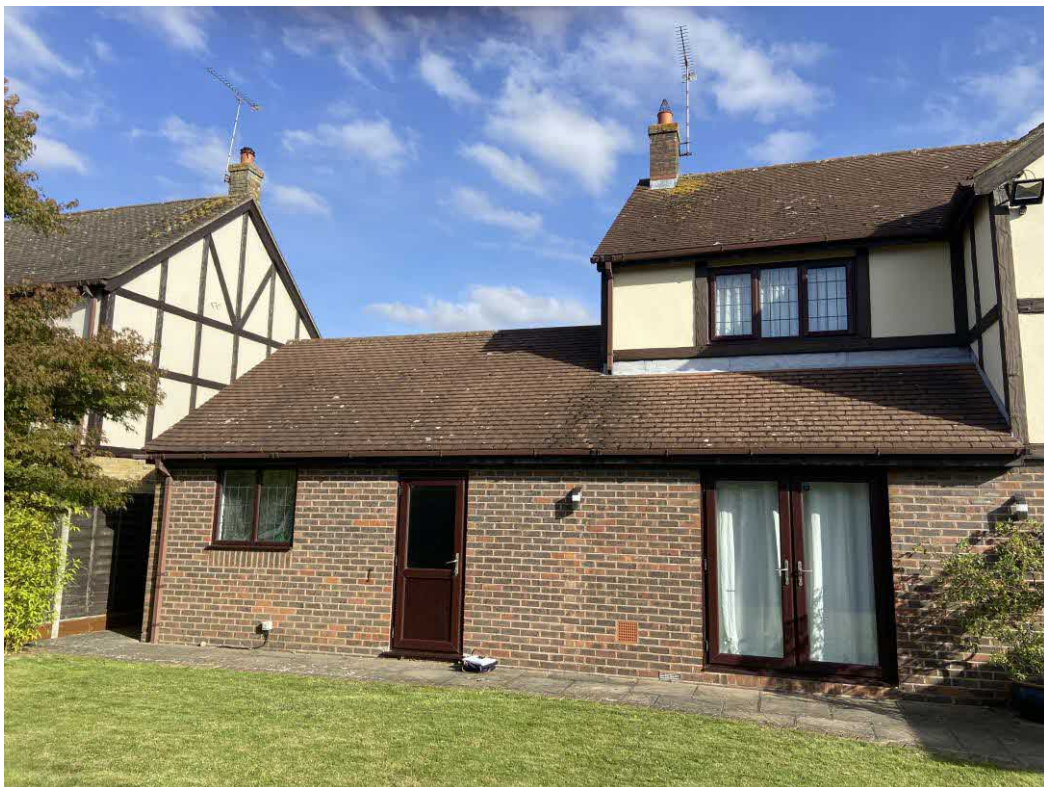
Rear elevation photo
