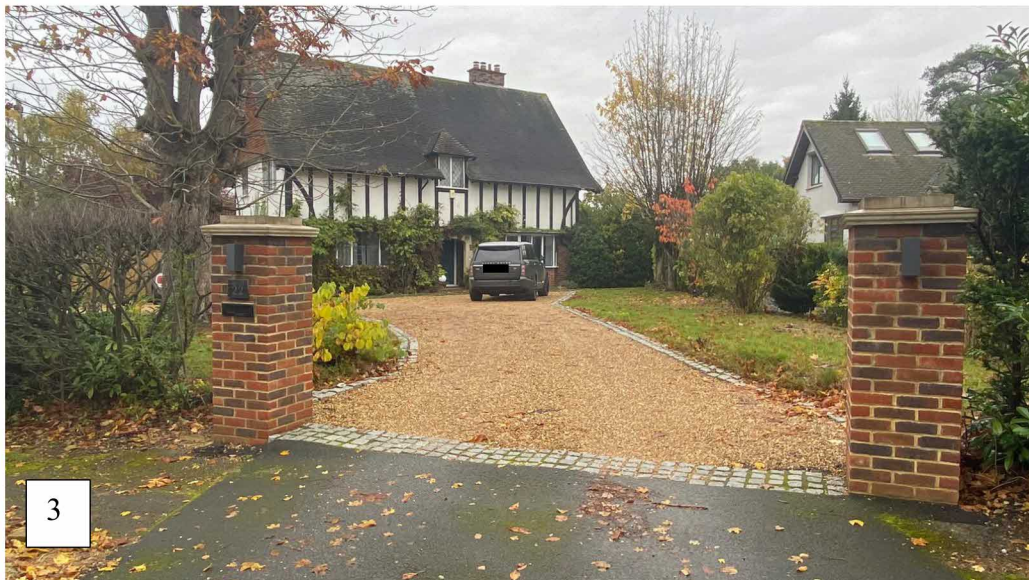
Fig 1: The Existing front façade of the house portrays a rusticated base with a timber framed white rendered First floor. (author)
