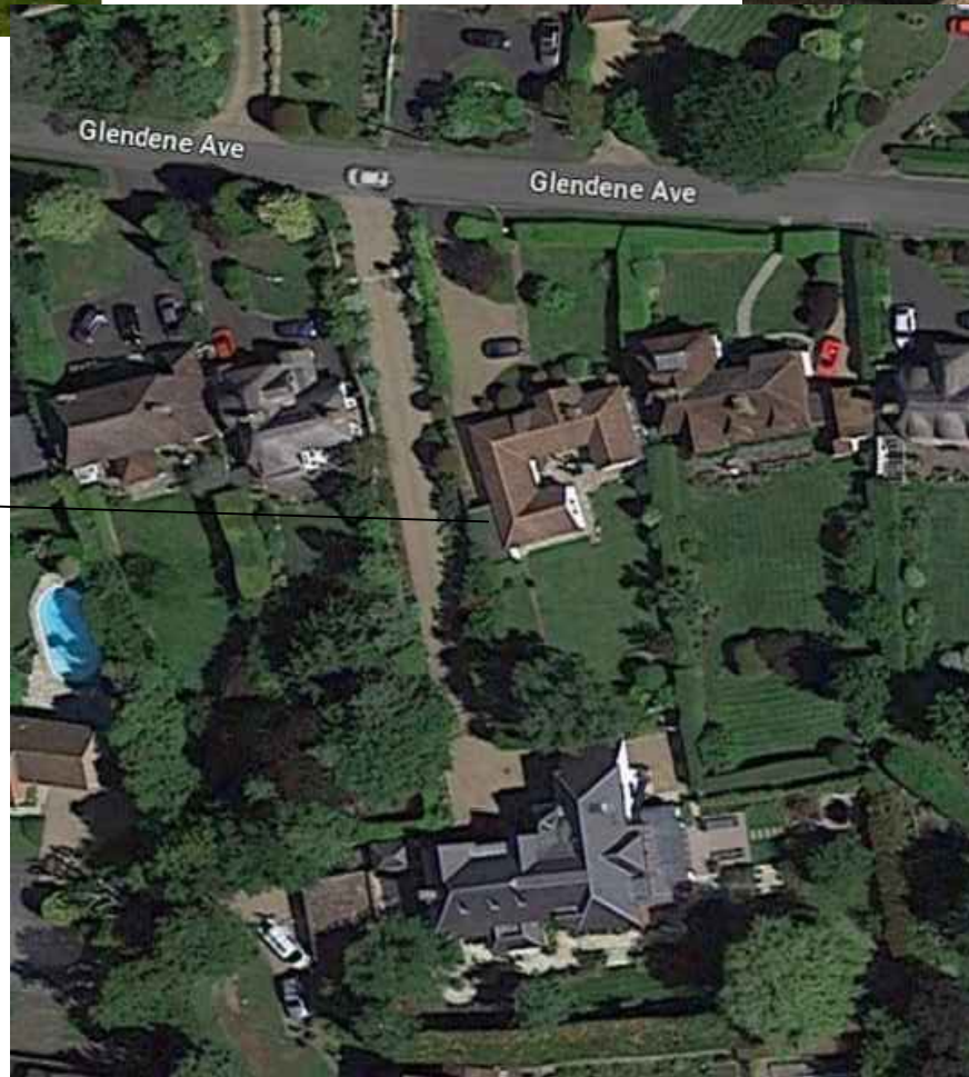
Overhead view of the bungalow showing the garage location and the relevant screening from neighbouring properties.
