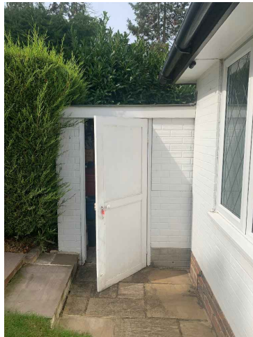
View of the side access door to the garage from the rear garden, ground rear to be reduced and retained with low level retaining wall.
