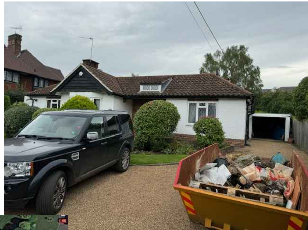
View of the front of the bungalow.
