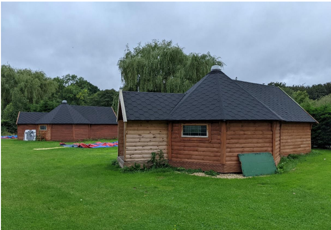
Photograph 1: Prefabricated timber cabins
