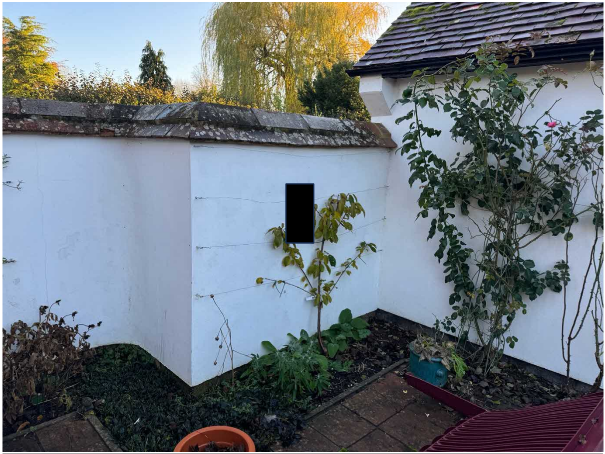
Photo 2 – Rear of wall
