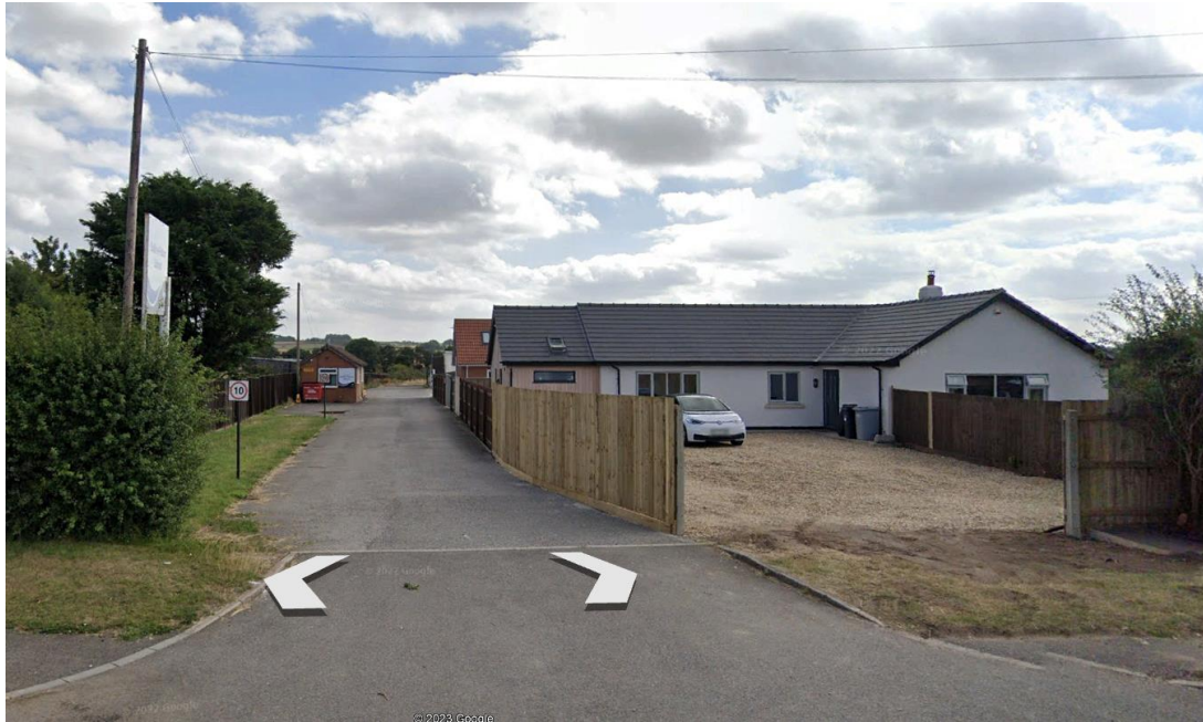
View of access to site from Horncastle Road
