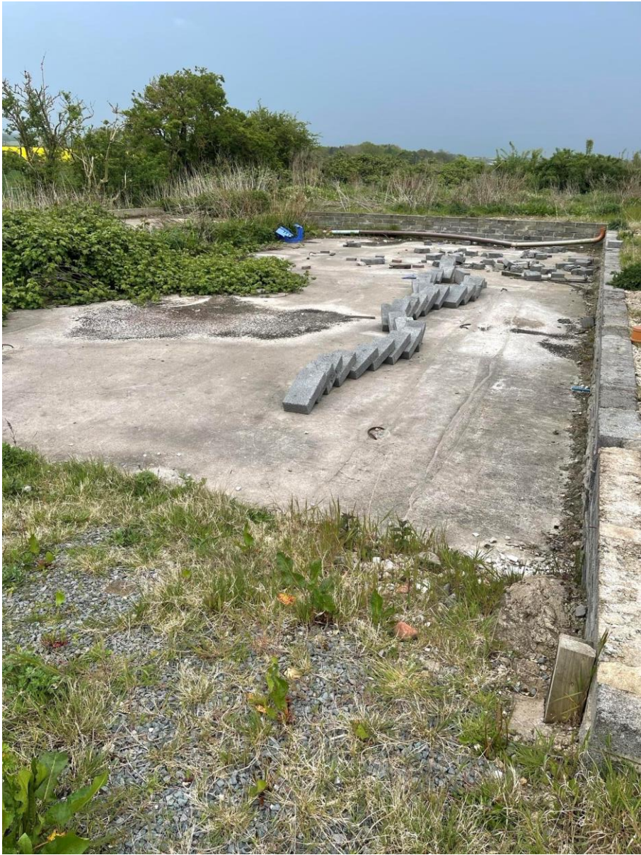
Photograph of hardstanding set at lower level
