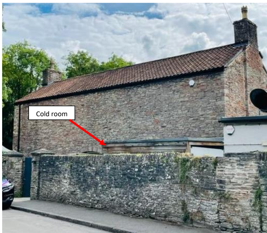
The external cold room as seen from the lane beside The White Horse
