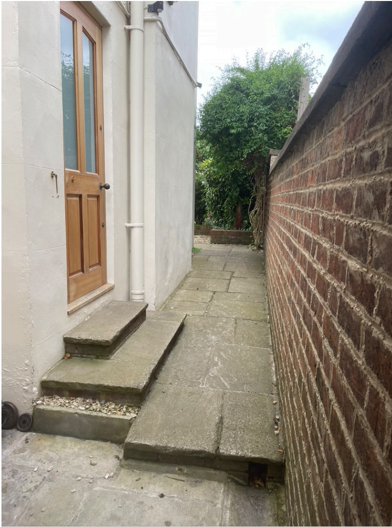
Picture of modern steps to be revised and modern doorway to be blocked
