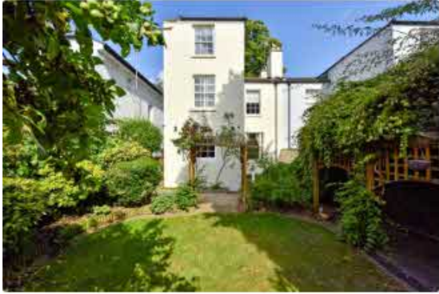
Rear Elevation no. 7 Sydenham Villas Road.
