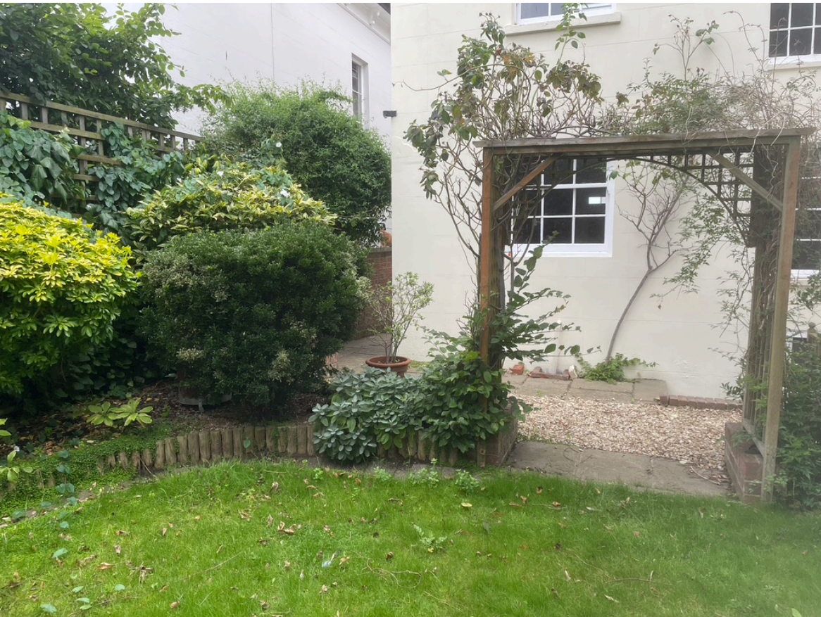
Picture of modern window to be replaced with new door with side lights
