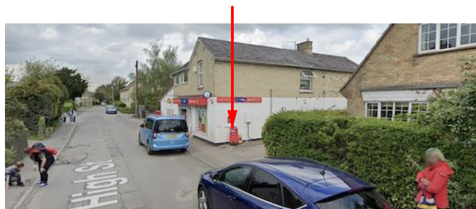
Existing access looking north, as proposed will remain unaltered
